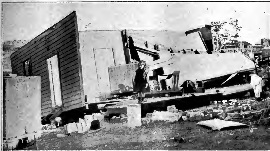
Another residence pushed off its foundations and partially demolished.
