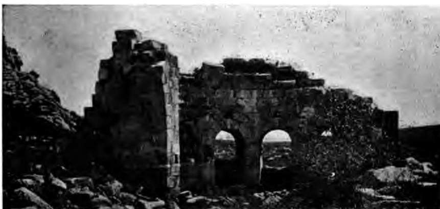
Fig. 6. — Interior of apse, northern basilica. Budrum.
