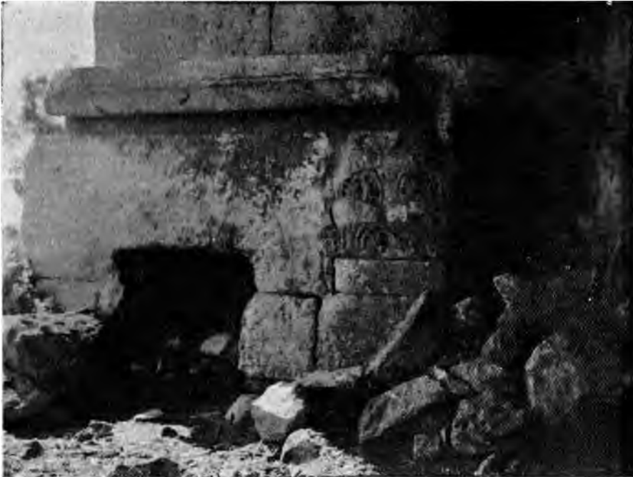
Fig. 5. — Ak Kale; south wall of eastern arm of cruciform; interior.
