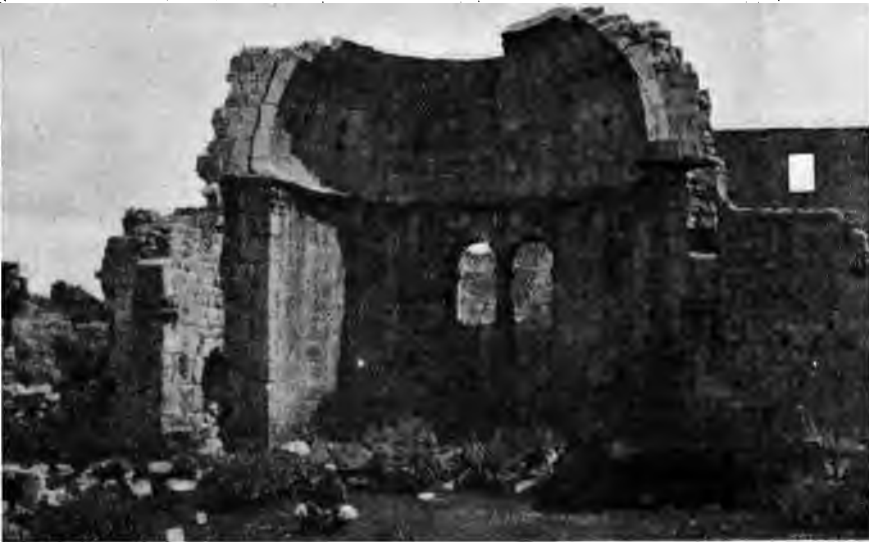
Fig. 14. — Kanytelideis, basilica No. 1, interior of apse.
