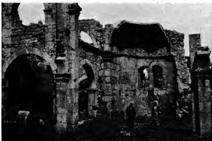
Fig. 25. — Kanytelideis; basilica No. 4, interior of apse.
