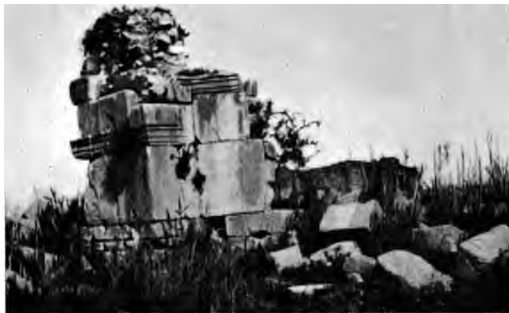
Fig. 10. — Basilica no. 1. Anazarbus. Exterior of apse, South-east angle.
