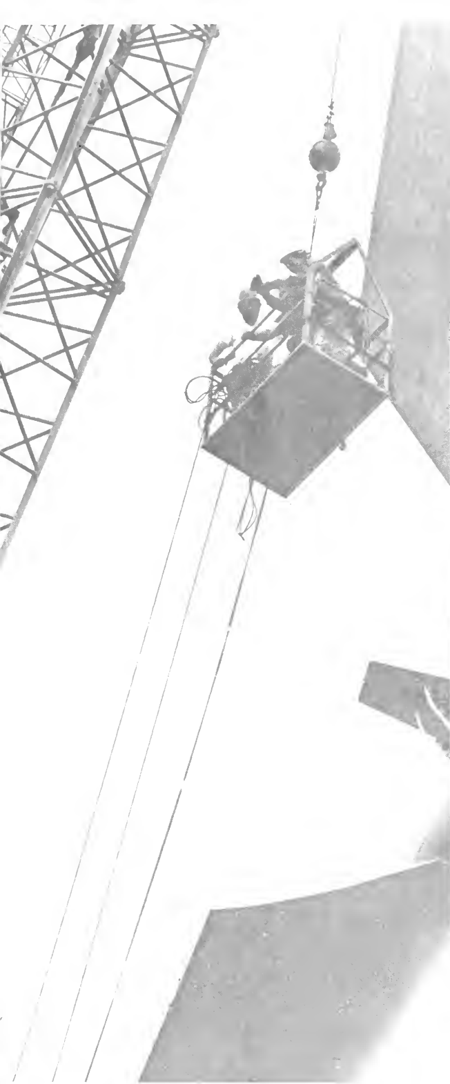
During the first few days of the 1983 fall semester, workmen came to Boone to dismantle the windmill. At top, the burning off of bolts to allow crane operators to lower the blade to the ground. Middle, one blade has been removed. Bottom, the first blade comes to rest on the ground.
