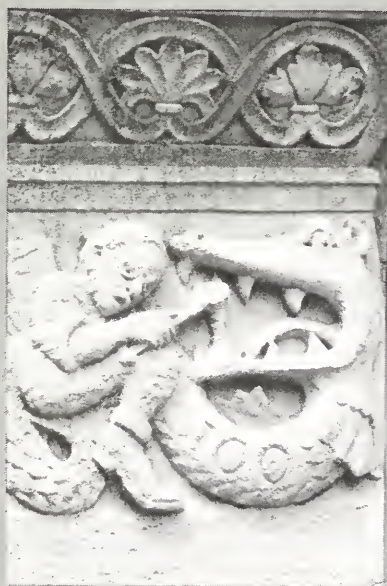
Cover photo: stone carving on capital of Chemistry Building of student extracting poison from dragon's mouth
