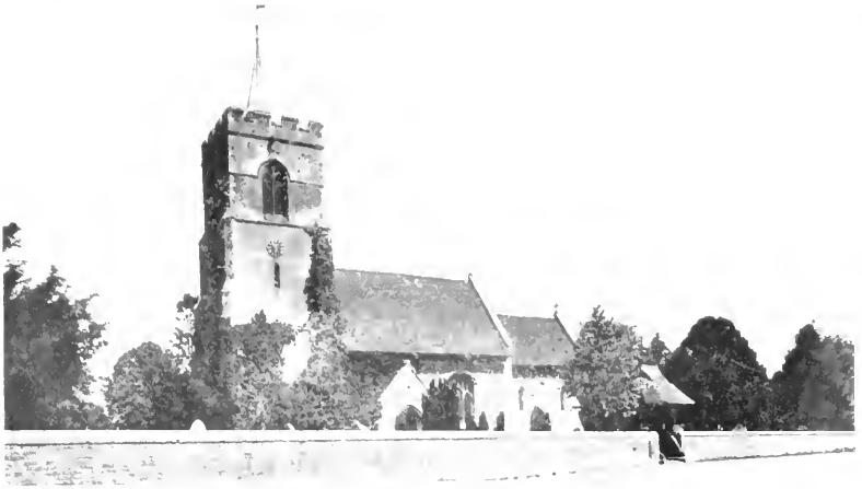
ST. MARY'S CHURCH, WEST MILL, HERTS.
