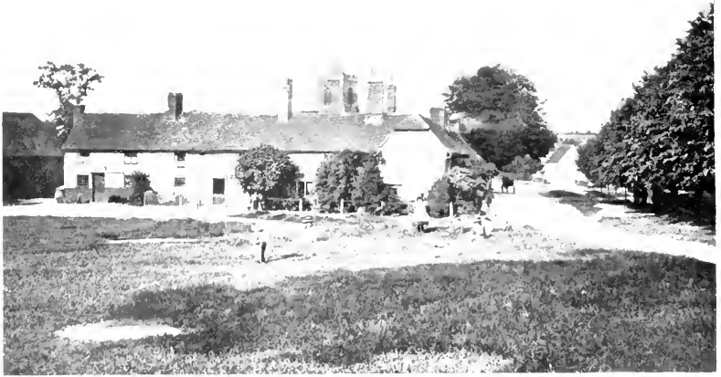
A VIEW OF WEST MILL, HERTS.
