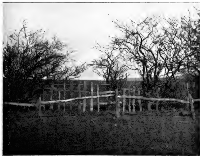
Fig. 235. Double posts and rails: rails about 3 ft. 6 in. high; and about 10 ft. apart.
