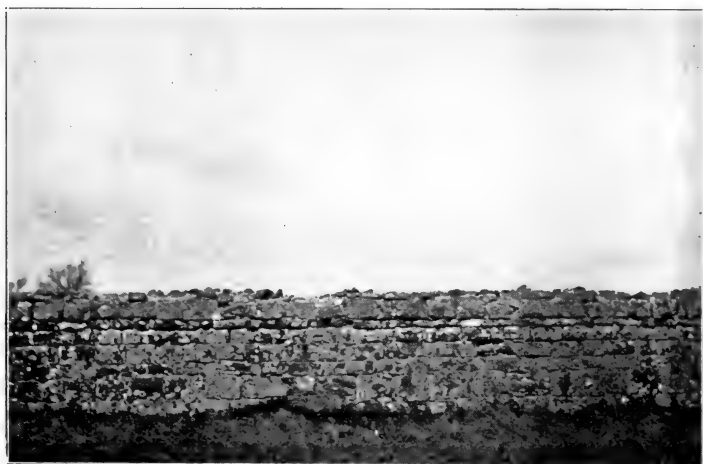
Fig. 238. Stone wall ; 4 ft. 6 in. high.
