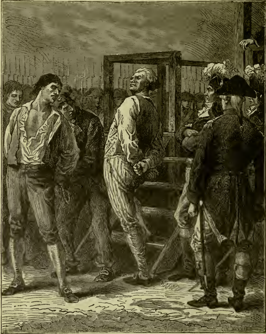
DANTON MOUNTING THE SCAFFOLD.
