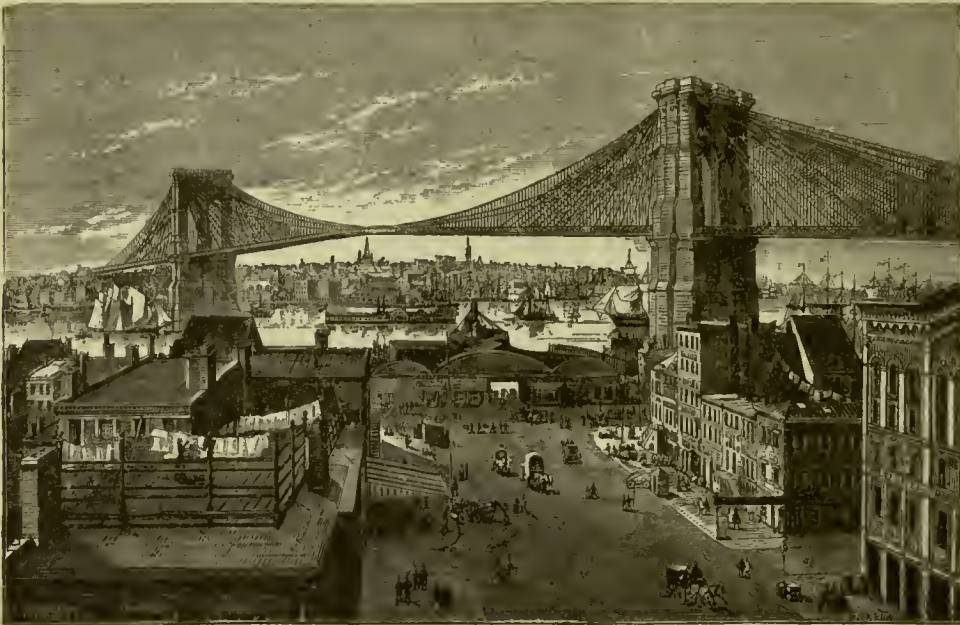
EAST RIVER BRIDGE, CONNECTING NEW YORK AND BROOKLYN.
