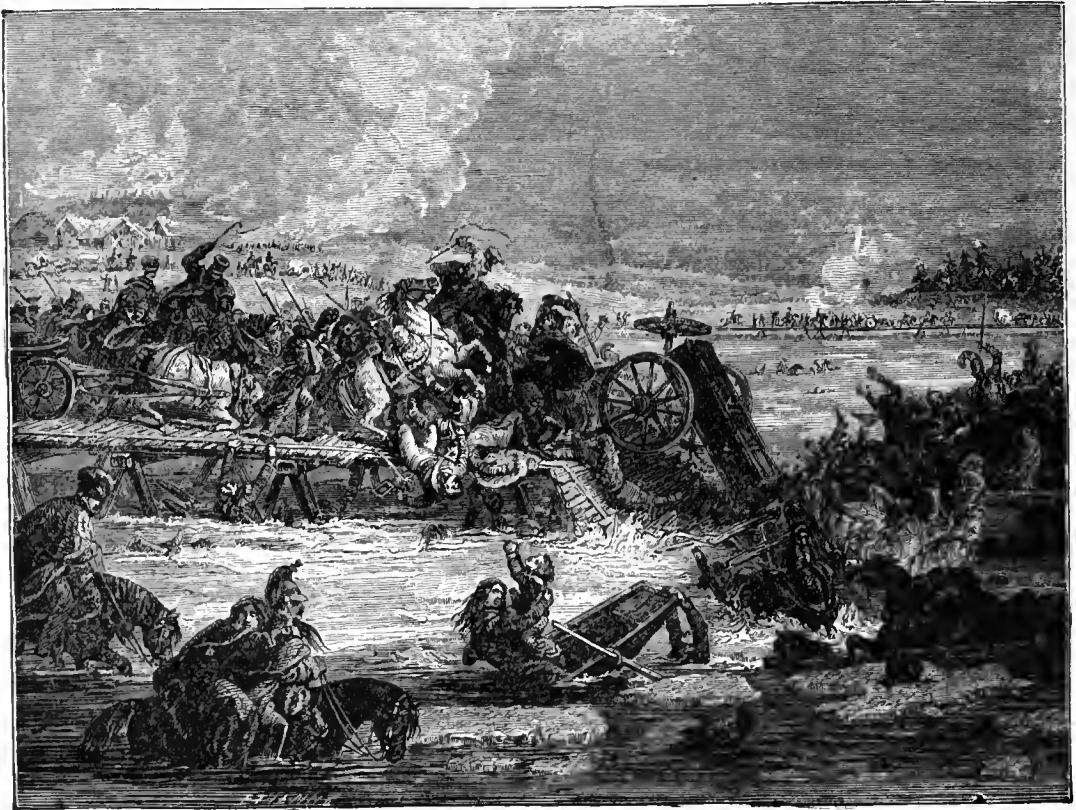
BREAKING DOWN OF THE BRIDGE AT BERESINA.
