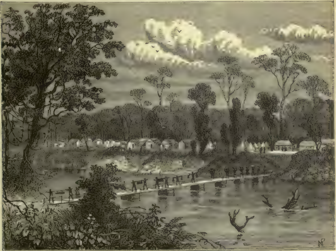
PONTOON BRIDGE OVER THE PRAH.
