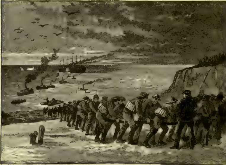
LANDING THE ATLANTIC CABLE.
