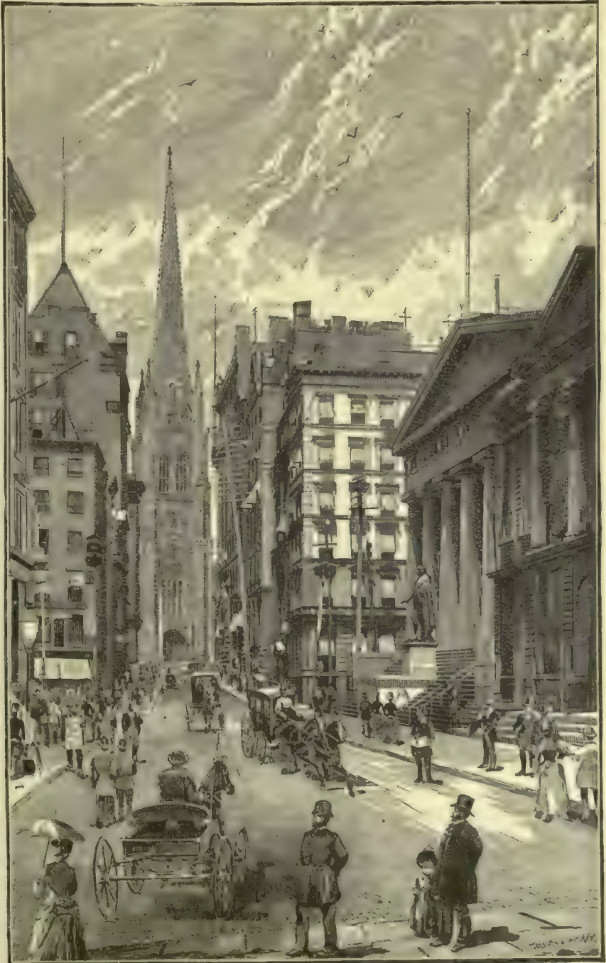
SUB-TREASURY BUILDING, WALL STREET.
