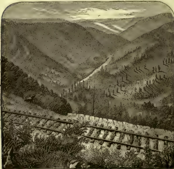
CENTRAL PACIFIC RAILWAY, SIERRA NEVADA.
