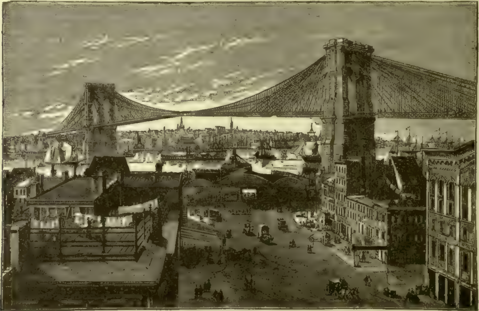
EAST RIVER BRIDGE.
