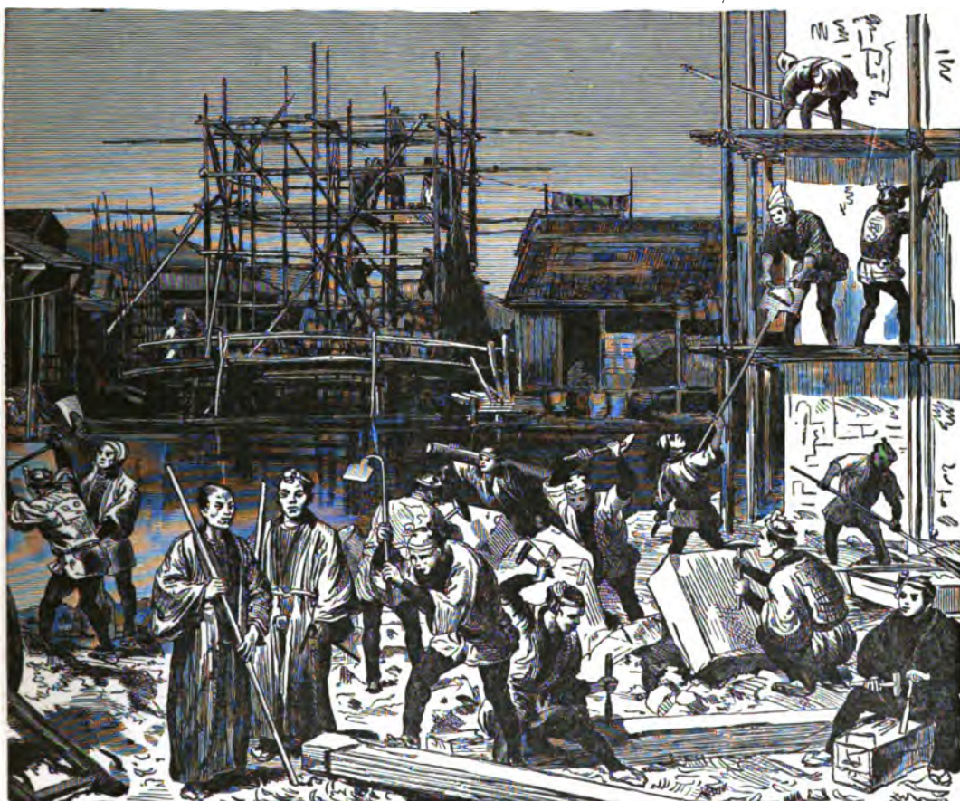
HOUSE BUILDING AT YOKOHAMA.—Drawn by L. Crepon, after a photograph.
