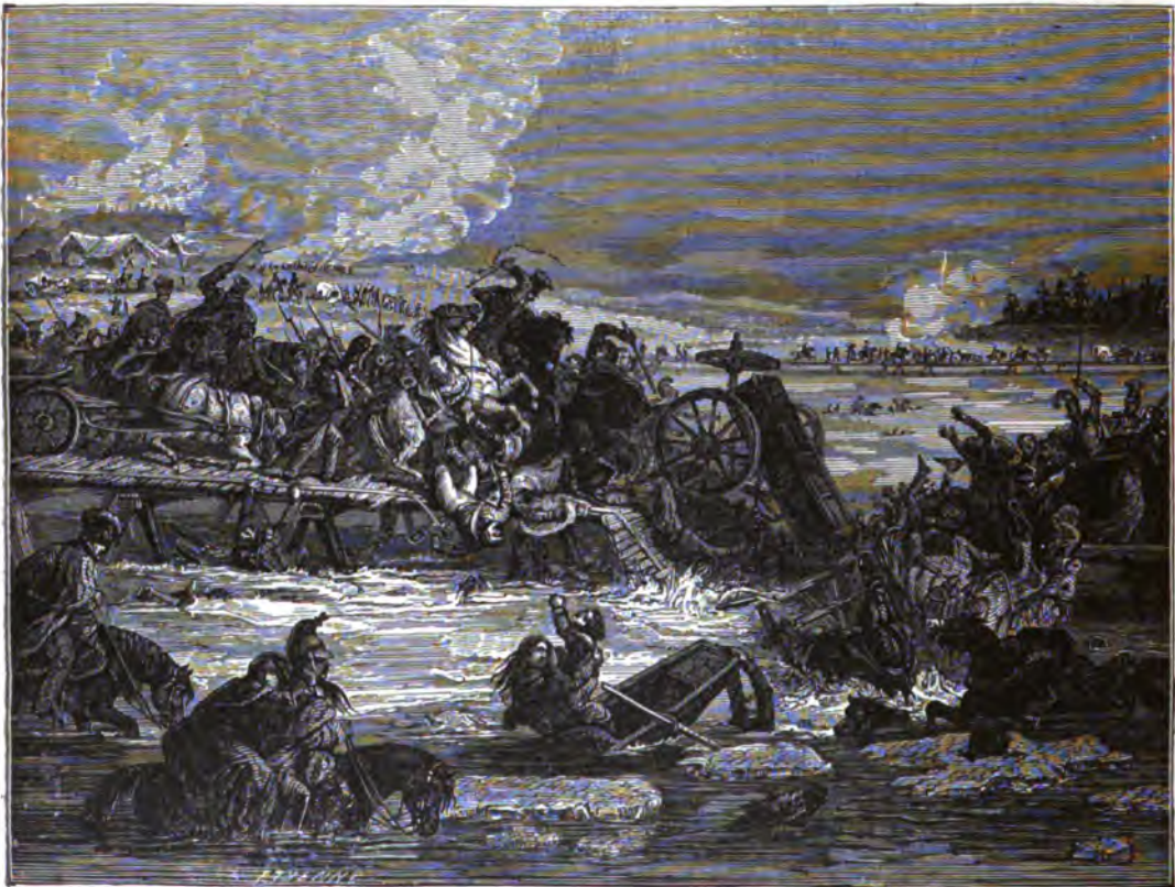
BREAKING DOWN OF THE BRIDGE AT BERESINA.
