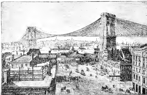
EAST RIVER BRIDGE
