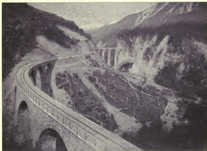
ONE OF THE INTERESTING SECTIONS OF THE RHÆTIAN RAILWAY IN THE CANTON OF THE GRISONS.
