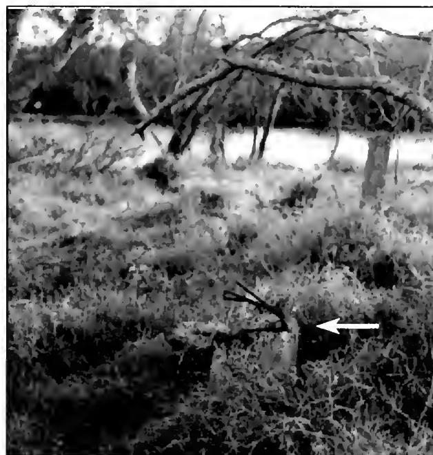
Figure 2-11: Example of concrete rubble found at several points along the north bank of the Nueces River downstream from the IH 37 bridge. It is speculated that this material was intentionally placed in low portions of the bank to reduce flooding of adjacent pastures and was probably acquired from the highway bridge renovation during the late 1950’s.
