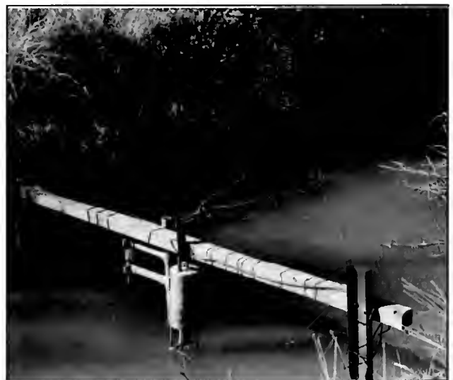
Figure 3-3: View of the Rincon gauge (Station 08211503).
