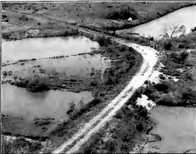
Figure 1-6: View of the private road crossing separating the upper and central Rincon Bayou channels. This pre-existing structure (constructed between September 1992 and March 1993) was not part of the demonstration project. The photo was taken on June 26, 1997, during the first significant flow event. During larger events, the structure backed water up in the upper Rincon Bayou (left), as indicated by the difference in water levels on either side of the road.
