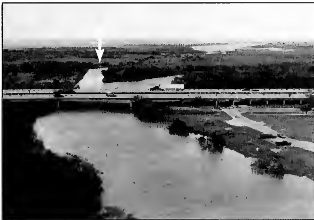
Figure 1-5: View of the Nueces Overflow Channel. The view is looking northeast, with the Nueces River in the foreground, and Rincon Bayou in the distant background. The photo was taken on June 26, 1997, during the first significant flow event.
