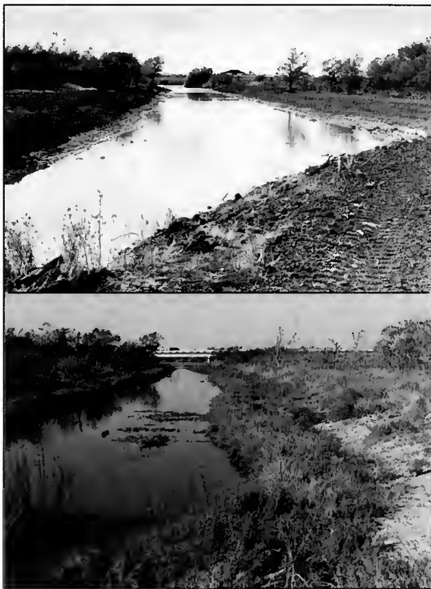
Figure 3-14: The Nueces Overflow Channel looking southwest. Note the changes in vegetation and channel characteristics from October 1995, immediately after construction (above), to June 1999, towards the end of the demonstration period (below).
