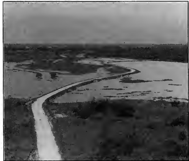
Figure 1-8: View of the low water crossing at the head of Rincon Bayou. This access road was one of several road improvements made as part of the demonstration project. The photo was taken on June 26, 1997, during the first significant flow event.
