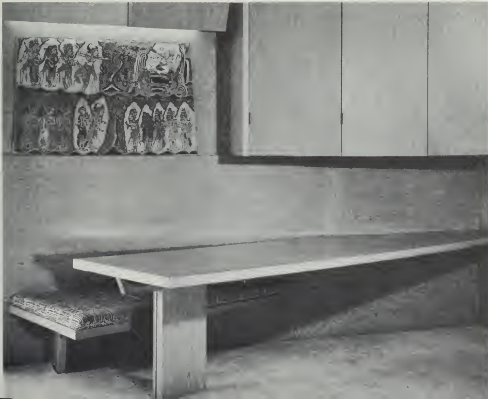
Remodeling of house for D. Gordon, Hollywood Hills, 1950 dining space (photo: L. Nossaman)
