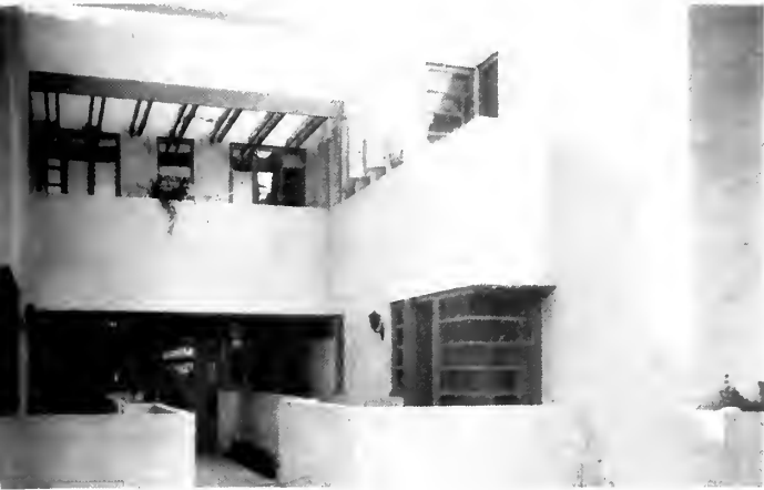
Apartment for S. Breacher, Los Angeles, 1925 (photo: V. Baker)
