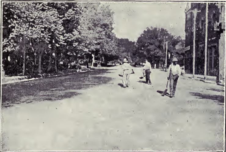
SPREADING SCREENINGS OVER TARVIA (Jackson, Tenn.).
