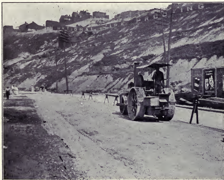
THE FINAL ROLLING. (Pittsburg, Pa.). TARVIATING.
