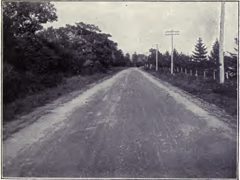
MERRICK ROAD, BETWEEN BELLMORE AND WANTAGH, L. I., N. Y. COLD APPLICATIONS OF TARVIA "B."
