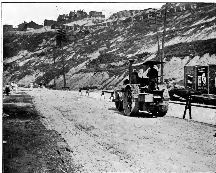
THE FINAL ROLLING. (Pittsburg, Pa.). TARVIATING.
