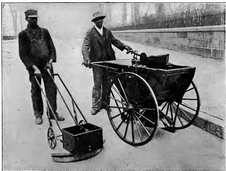
FLUSH COAT SPREADING MACHINE. (Patented.)
