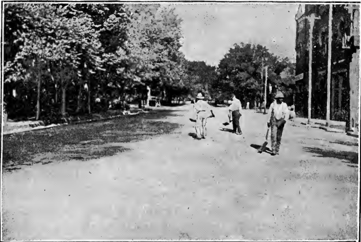
SPREADING SCREENINGS OVER TARVIA (Jackson, Tenn.).
