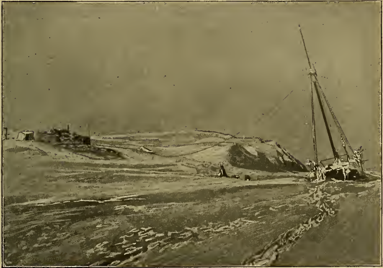
Kunak's House. Sten's House.
