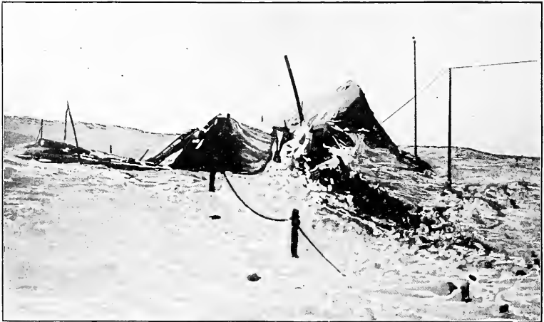
OUR RESIDENCE AT KING POINT
