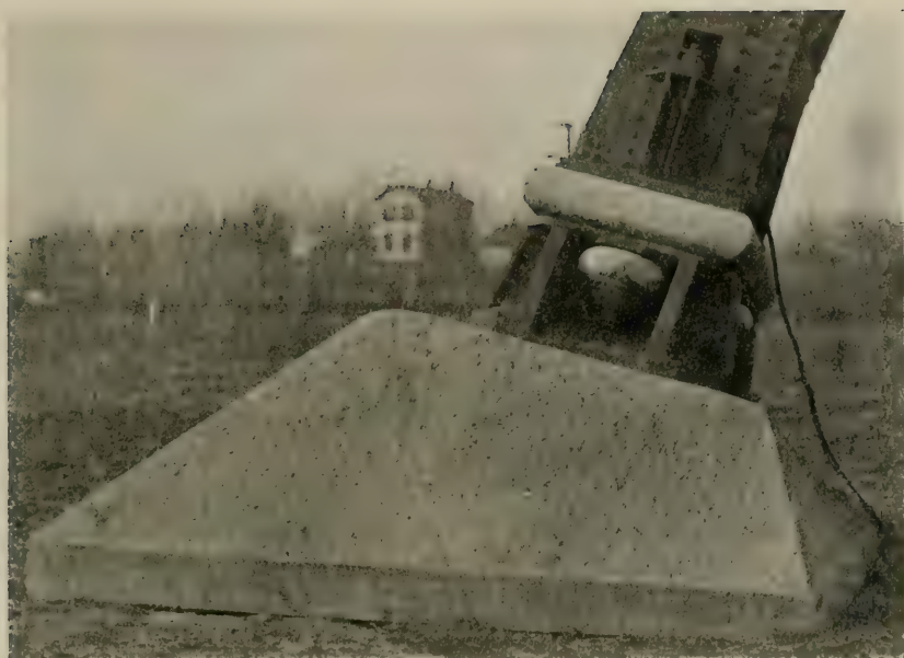
FIG. 97c.—Insulation at Base of One Leg of Tower.
