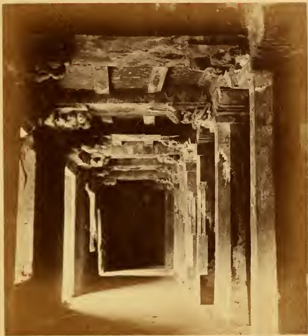
AISLE IN HALL OF VIHARA No. 17.—AJUNTA.
