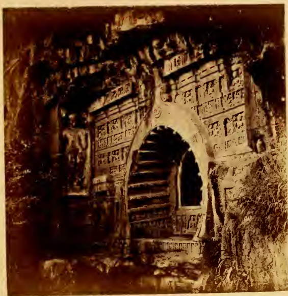
UPPER PART OF FACADE, No. 26.—AJUNTA.
