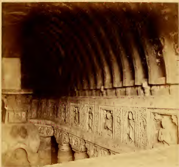
ROOF OF CHAITYA, No. 19.—AJUNTA.
