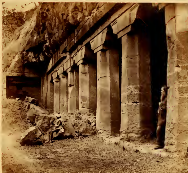
FACADE OF CAVE No. 4.—AJUNTA.
