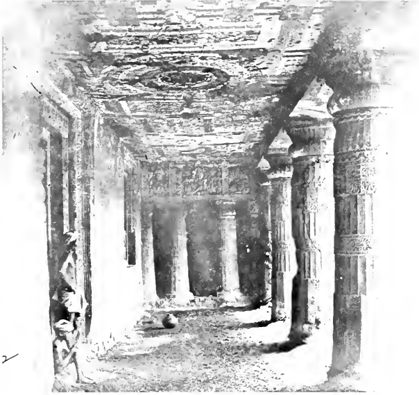
VERANDAH, CAVE No. 2.—AJANTA.
