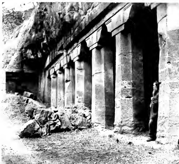
FACADE OF CAVE No. 4 - AJUNTA
