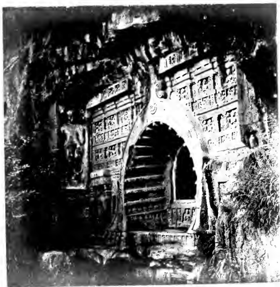
UPPER PART OF FACADE, No. 26.—AJUNTA.
