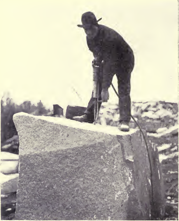
Fig. 37. Method of Using Hammer Drill.
