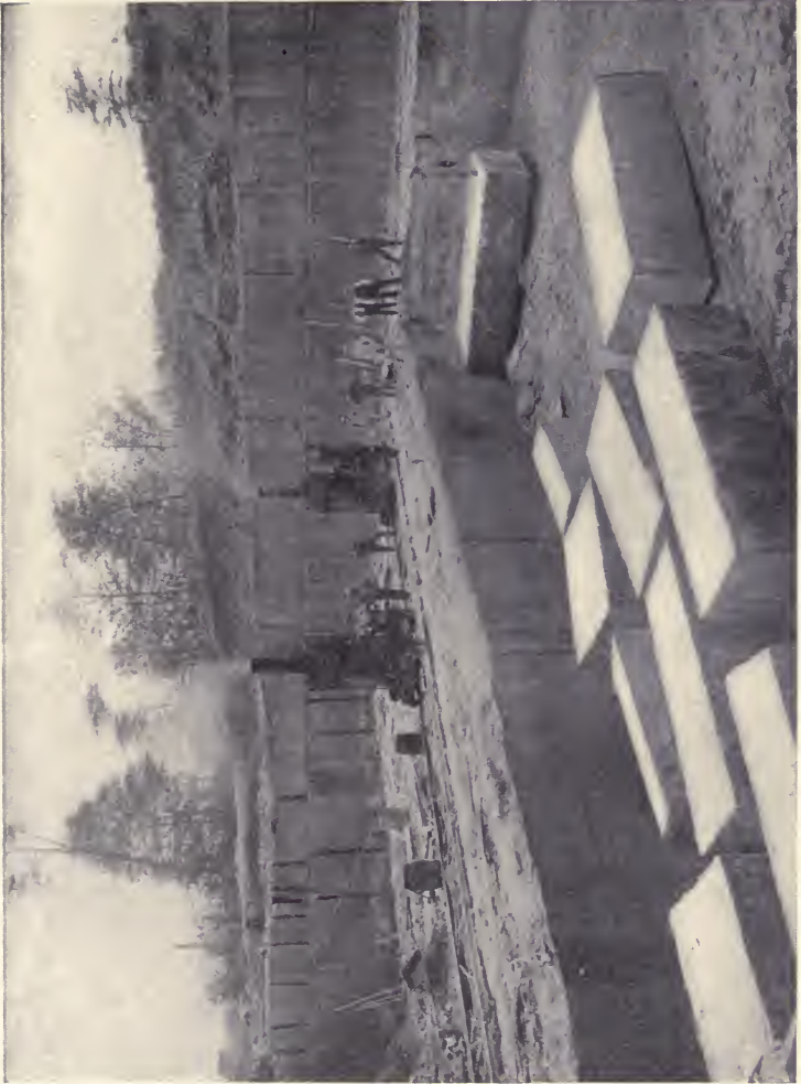
Fig. 45. Quarrying Dimension Stones with Channeler.
