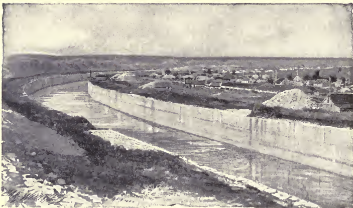
Fig. 44. Channeled Walls of Chicago Drainage Canal.
