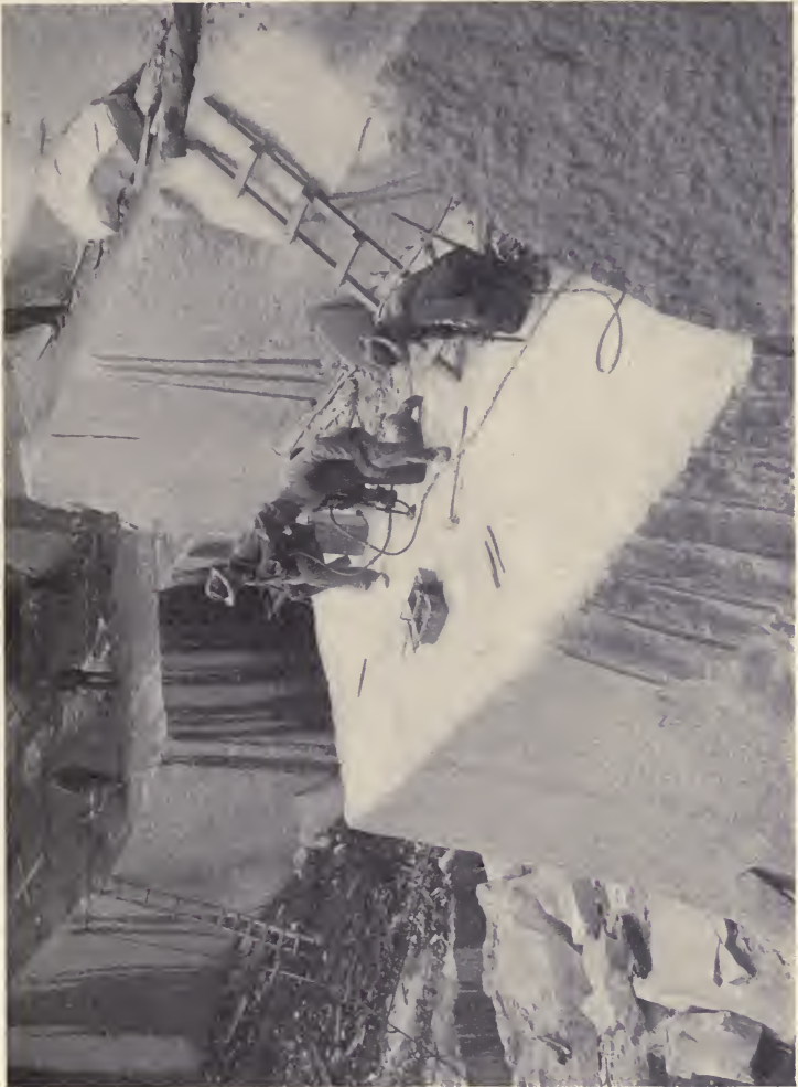
Fig. 6. Regular Bench Work in a Quarry. At Work with Drills.
