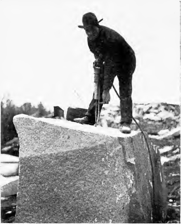
Fig. 37. Method of Using Hammer Drill.
