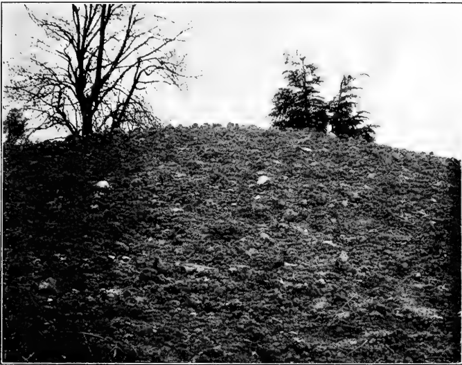
THE BANK. (Roughly formed before rocks are put into place.)
