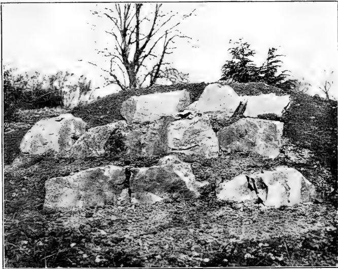
ROCKWORK ADVANCING UP THE HILL.
