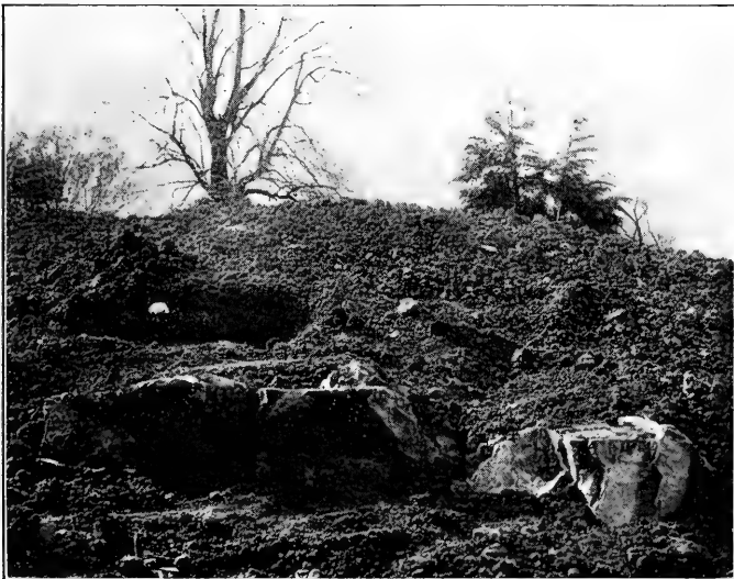
FIRST LINE OF ROCKS LAID.
