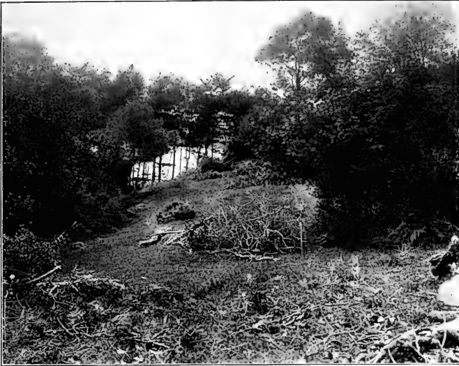
BANK TYPE. (Site being cleared.)
