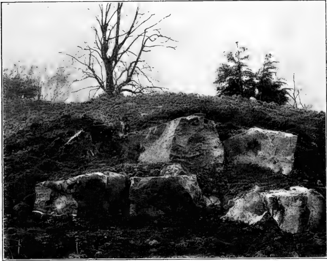
SECOND LINE OF ROCKS IN POSITION.
