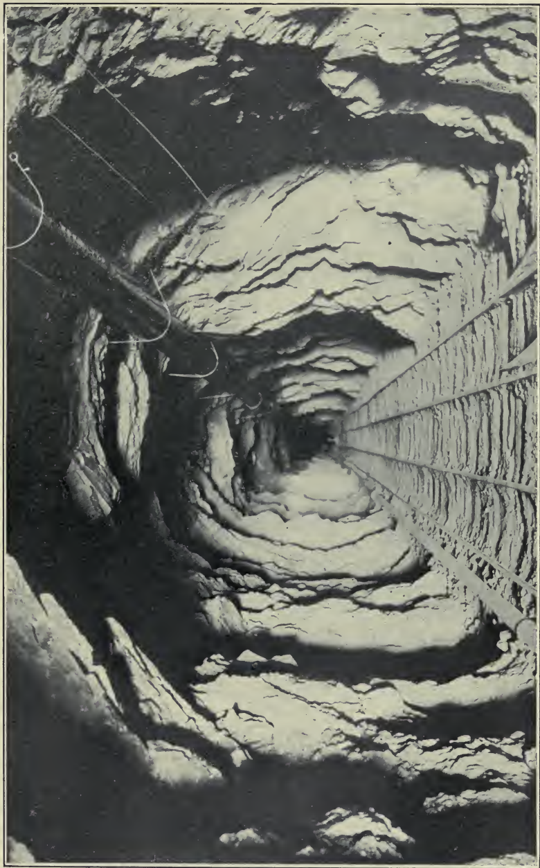
A double track drainage and transportation tunnel. The small pin point of white is day light at the portals.
