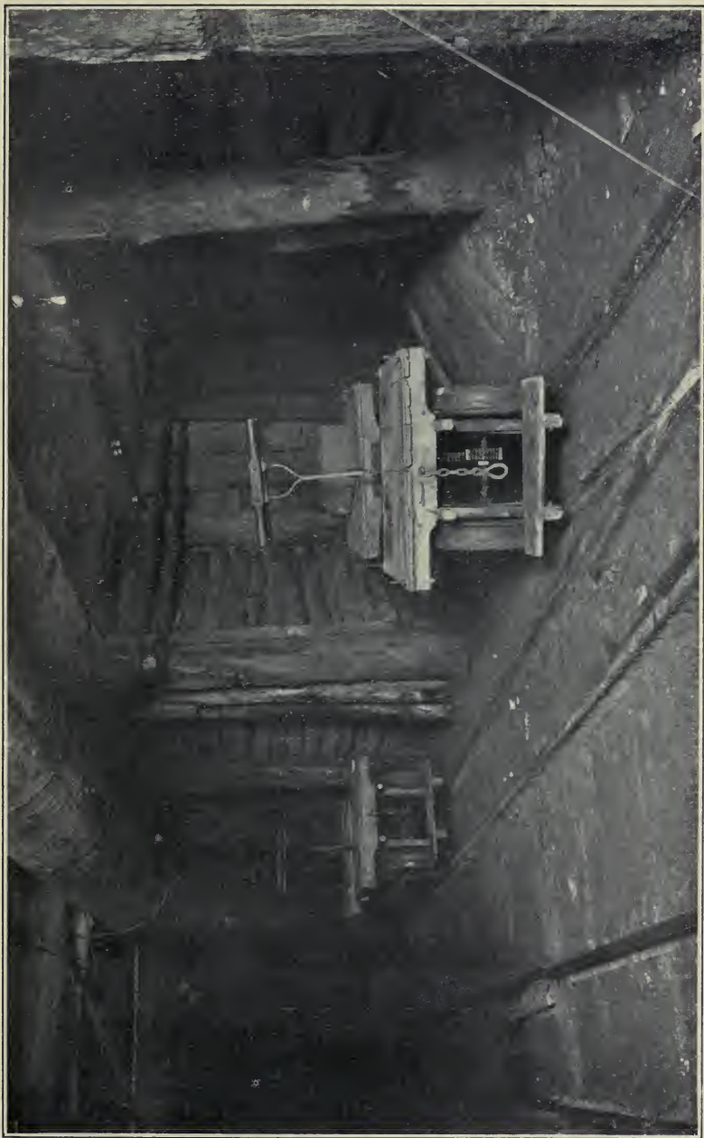
Point of intersection of a vein by a cross cut tunnel. This point is 8,000 feet from the surface on the level, and 2,000 feet below the apex of the vein. Here the author wrote the last lines of this book.
