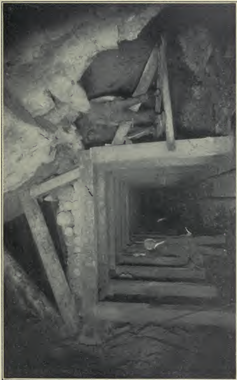
Timbering in a vein that dips from the perpendicular. The two miners are upon the hanging wall side of the vein.
