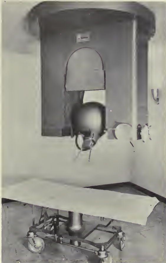
Fig. 5—Ceiling-mounted cobalt apparatus.
