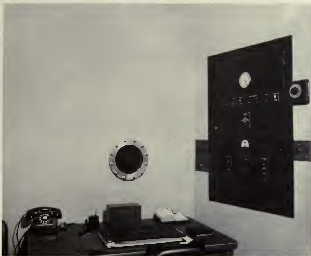
Fig. 1—Control panel, showing switches for moving radium ring, water window for observation of patient through concrete wall 2 ft thick, and speaking system for communication with patient.
