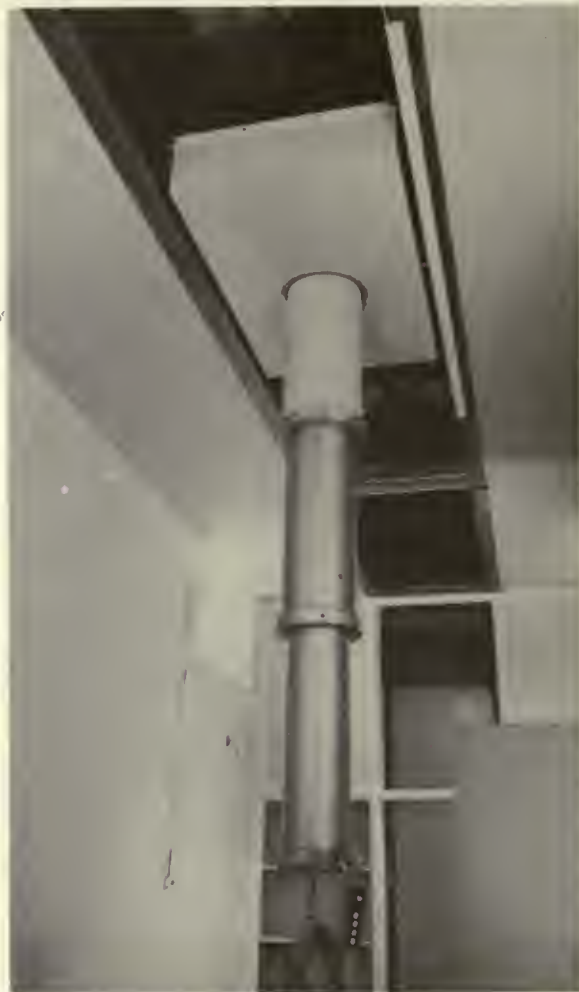
Fig. 10—Stabilatron II ceiling mounting.
