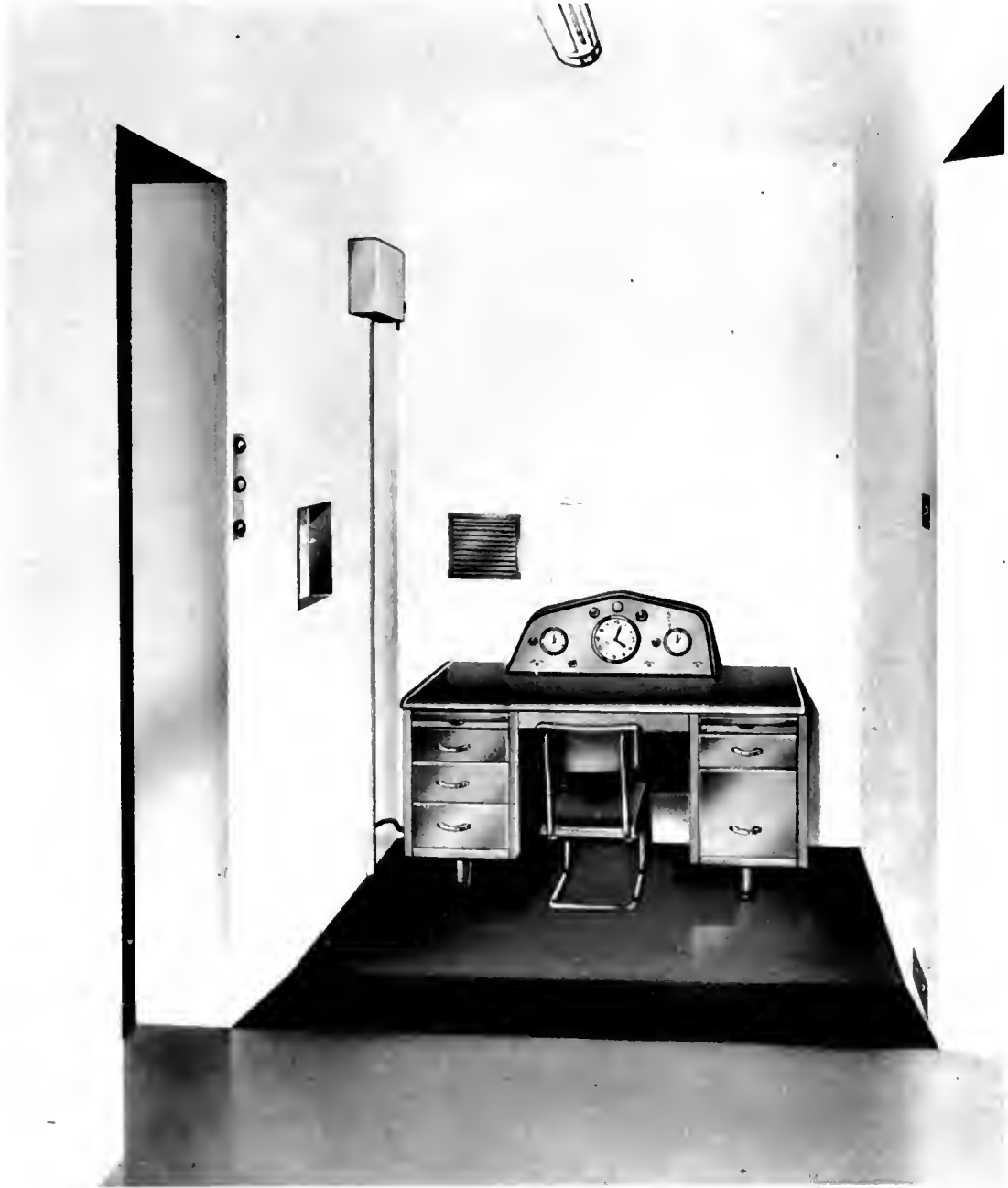
Fig. 3—Cobaltron remote-control panel.
