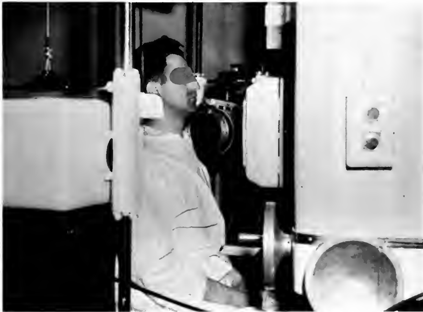
Fig. 5—Patient set up for treatment of carcinoma of the thyroid gland by cobalt rotation therapy. The 140-kv X-ray diagnostic unit is seen at the patient's left shoulder, and the image-intensifier fluoroscope is seen at the patient's right shoulder.
