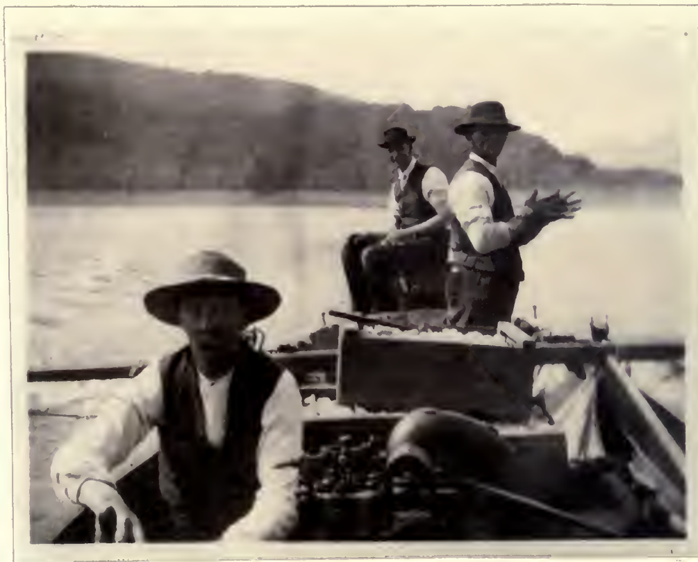
COPPER SULPHATE TREATMENT AT LAKE CHABOT
