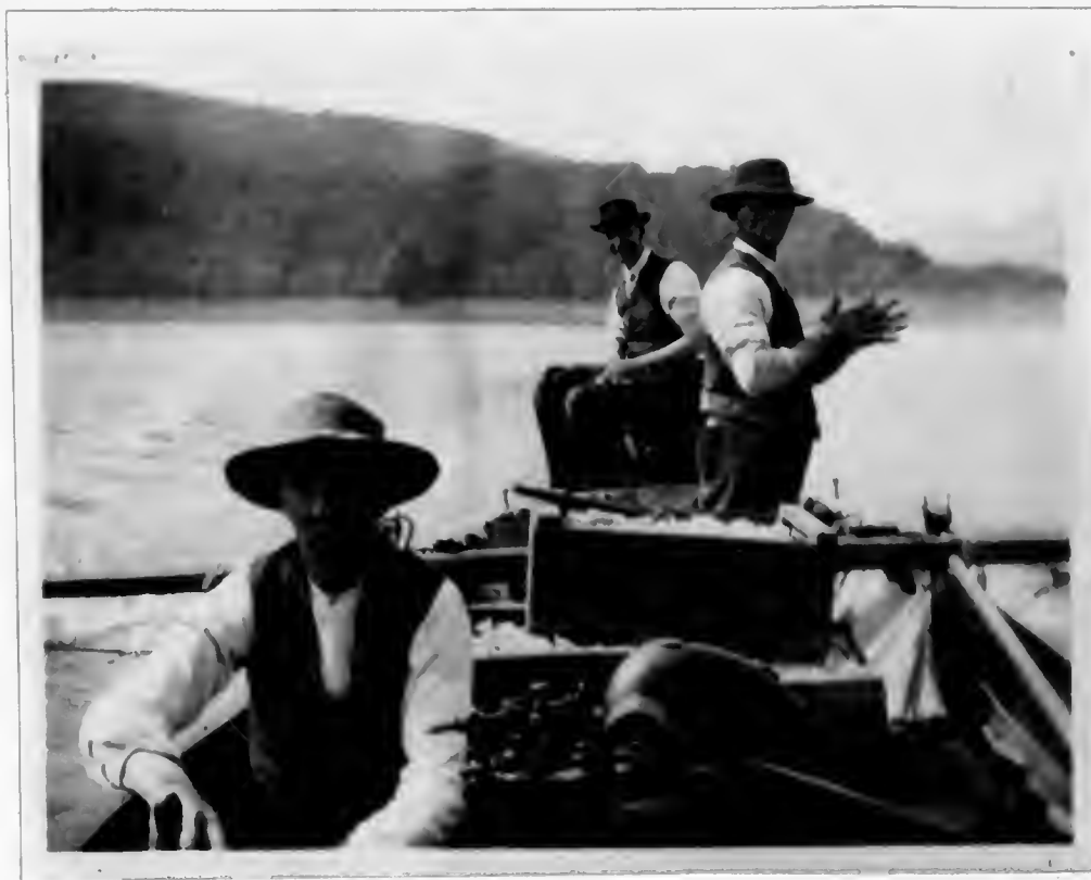
COPPER SULPHATE TREATMENT AT LAKE CHABOT
