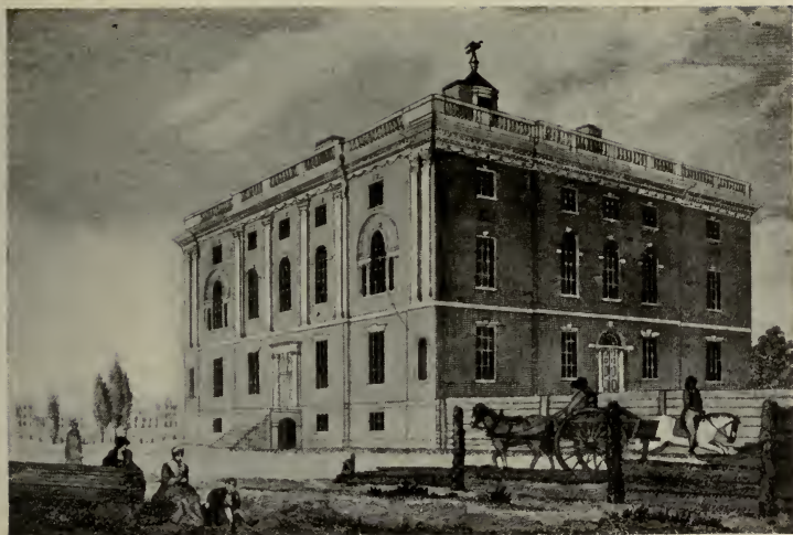
THE HOUSE INTENDED FOR THE PRESIDENT OF THE UNITED STATES, ON NINTH STREET (From the engraving by Birch)
