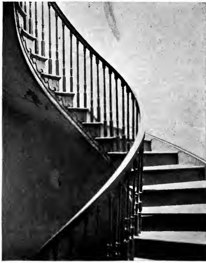
STAIRWAY AT 247 SOUTH SIXTH STREET
