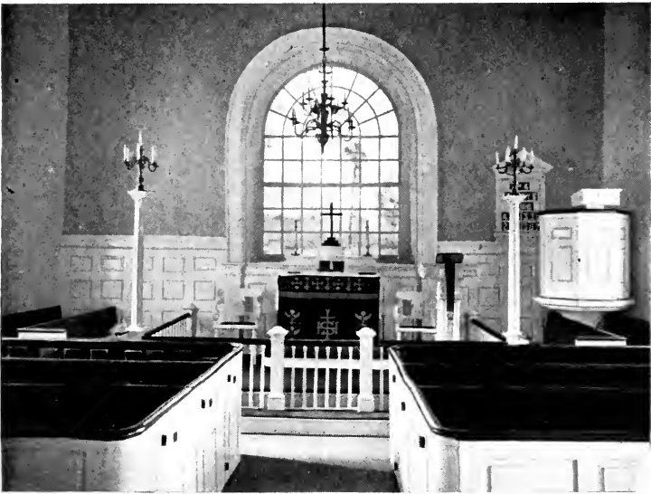
INTERIOR OF OLD ST. DAVID'S CHURCH, RADNOR
