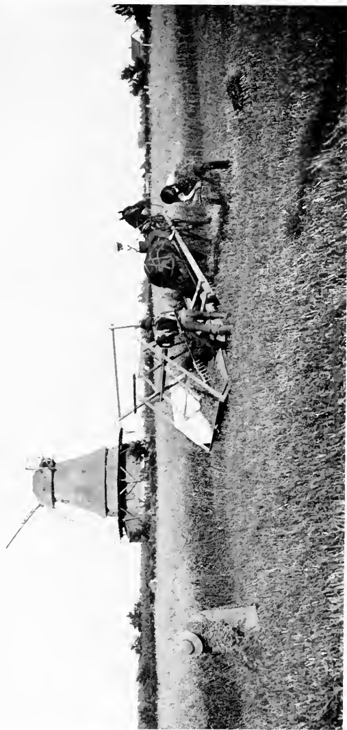
A MODEL OF THE FIRST PRACTICAL REAPER
