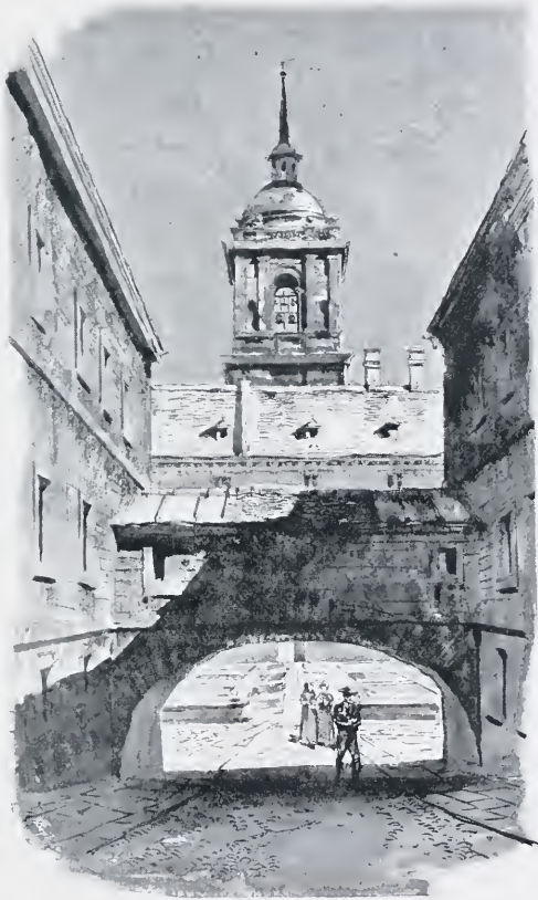
ARCHWAY LEADING TO THE ESCORIAL, AS SEEN FROM THE INN.
