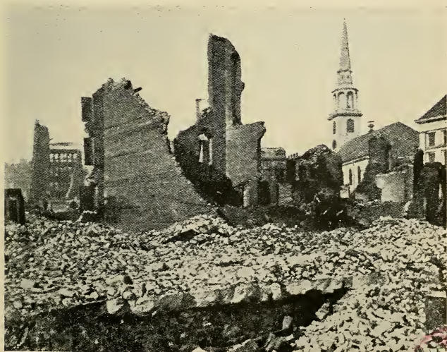
ANOTHER VIEW OF THE FIRE RUINS.
