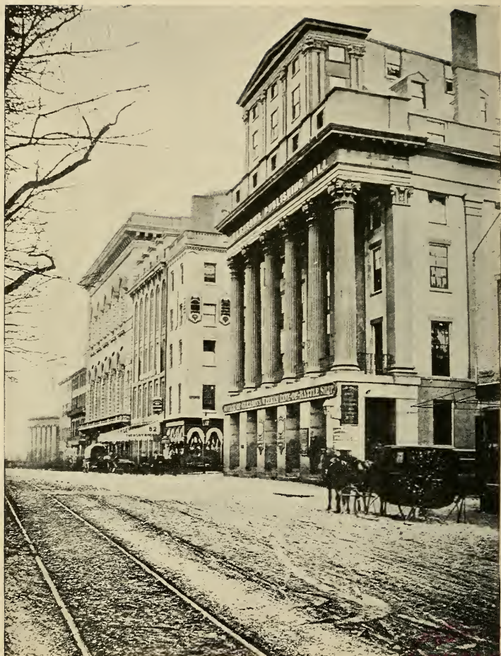
CORNER OF TREMONT AND BROMFIELD STREETS ABOUT 1870.
