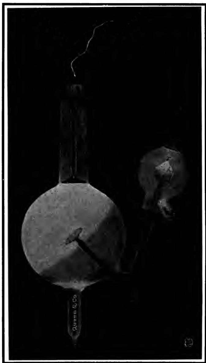
SELF-REGULATING X-RAY TUBE. OPERATING PROPERLY.
