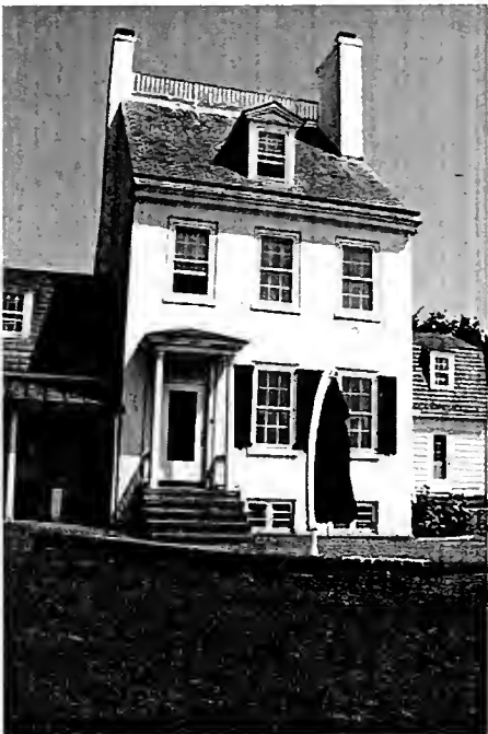
Figure 7 View of 1837 Addition from the South
