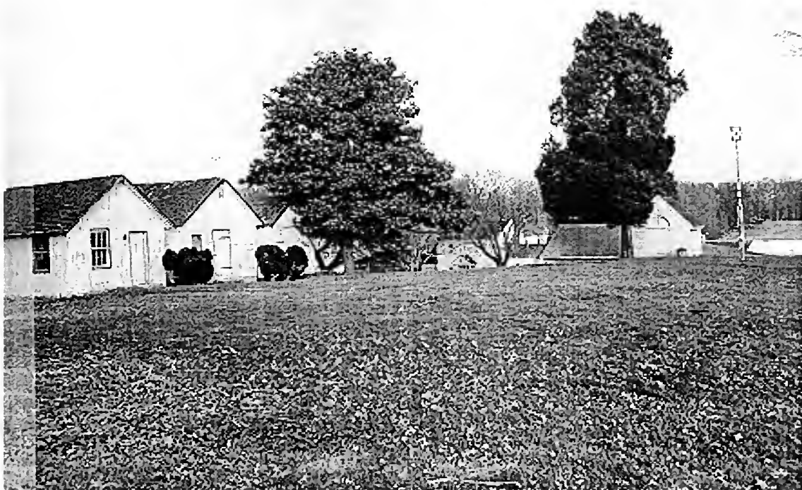
Figure 8 Outbuildings East of Main House
