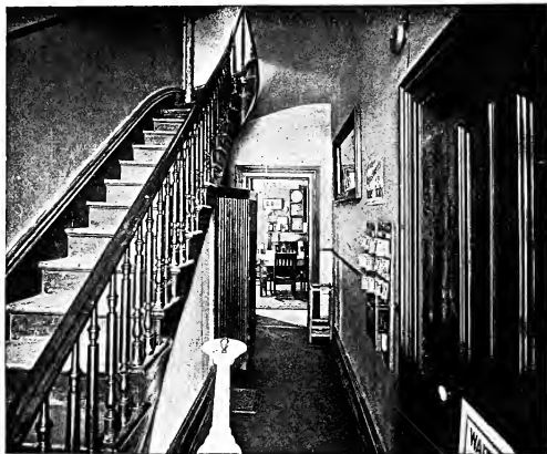
Clinic Entrance, Stairway Leading to Demonstration Rooms
