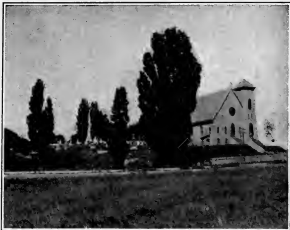
Church built with Stones taken from Fort Erie.
