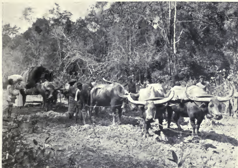
ARRIVAL OF MACHINERY AT KABIN.
