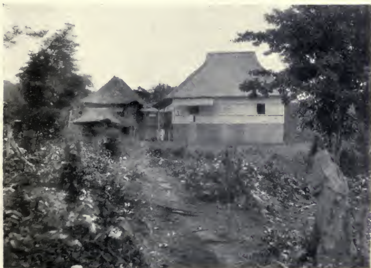
LONGOS MINE, BUNGALOW.
