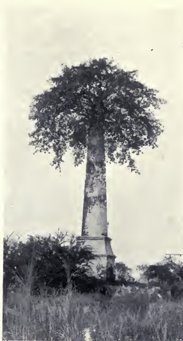
TREE GROWING IN CHIMNEY AT PECHIM.
