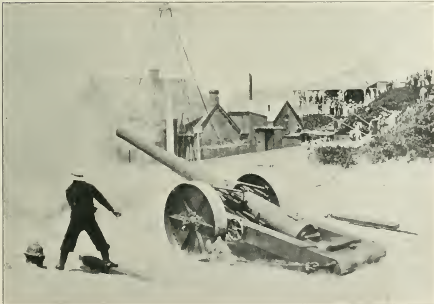
6 IN. Q-F. GUN, ON SCOTT'S MOUNTING.
