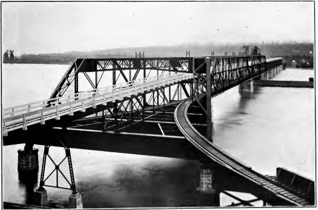
Bridge over the Fraser River at New Westminster, B.C., built by the DOMINION BRIDGE CO., LTD. for the British Columbia Government.
