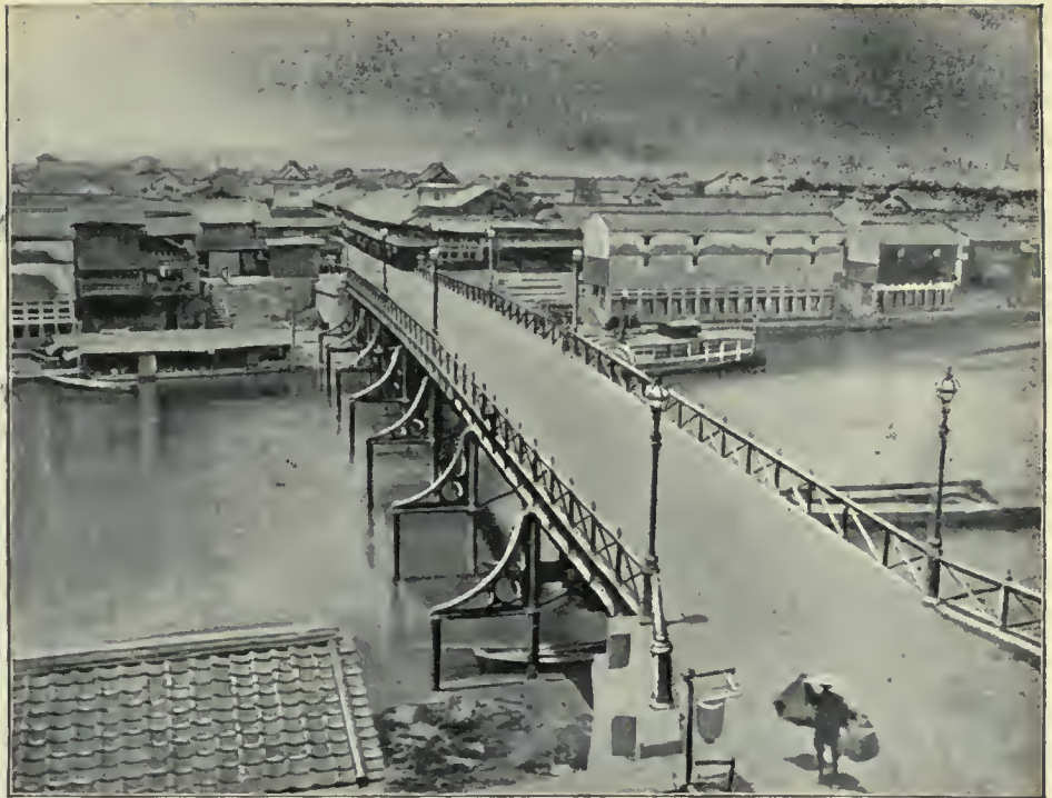
THE "KORIA BASHI" (COREA BRIDGE), OSAKA, JAPAN.
