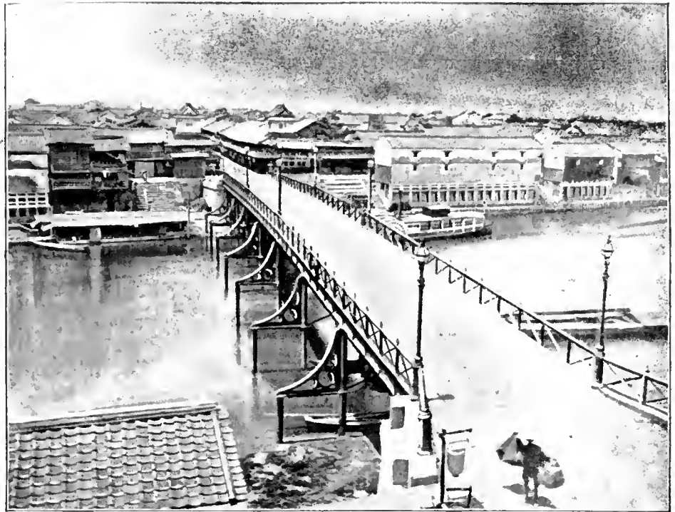
THE "KORIASASHI" (COREA BRIDGE), OSAKA, JAPAN.
