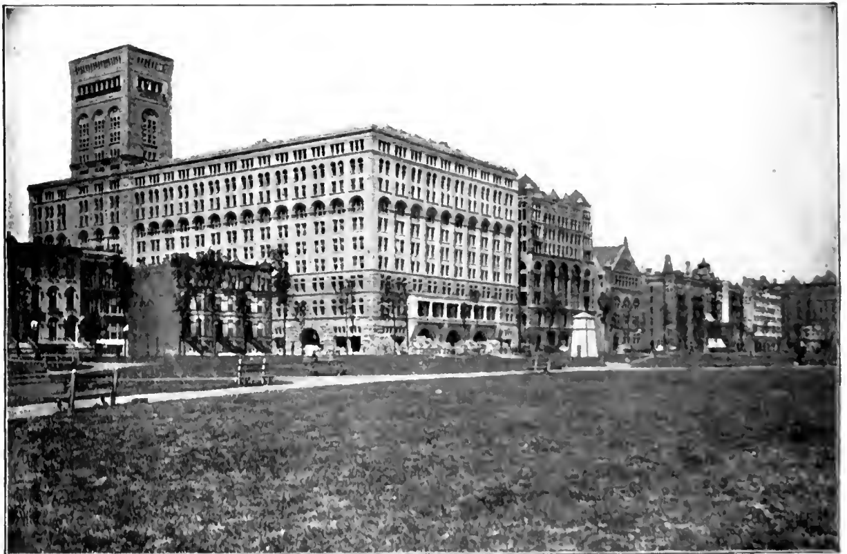
AUDITORIUM HOTEL, ON MICHIGAN AVENUE, CHICAGO. —This is one of the largest hotels in this or any other country, and will, no doubt, attract quite as much attention as the exhibits within the inclosure of the Fair grounds. It is thoroughly fire-proof; it contains all the latest modern improvements; is furnished with the costliest parlor, dining-room and chamber furniture, and is the equal, if not the superior, of the hotels in any city of the Union.
