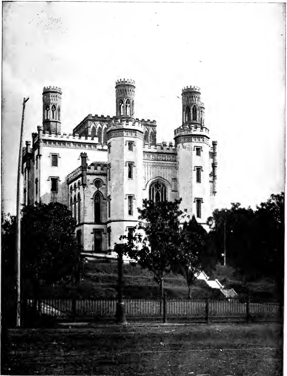
STATE CAPITOL, BATON ROUGE, LOUISIANA. —This very striking picture presents one of the finest specimens of architecture in the State of Louisiana. It is that of the State Capitol at Baton Rouge. The order of architecture is not decided, but it is one of those ho'd castellated effects which becomes the elevation on which it is erected. Since the entire city is built on a bluff, and the capitol on an elevation within the city, its situation is especially attractive. The city is 120 miles above New Orleans and on the Mississippi River. It was one of the first settlements of the French on the banks of the great river, and between it and New Orleans the rivalry for the honors of the capital site was long and earnest.
