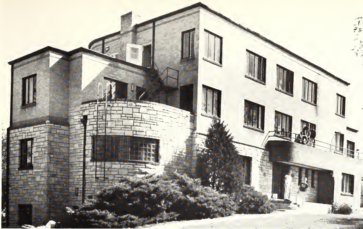
Housing at 508 Sunset features balconies both in the front and back. Phi Delta plans are to pave part of the parking lot during the summer for a recreation area.
