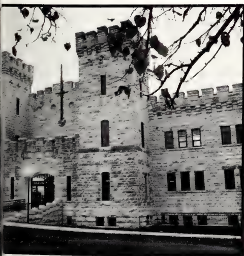
Nearly 17 years after the interior of Nichols Gymnasium was destroyed, the renovated structure was officially rededicated on Nov. 16, 1985.
