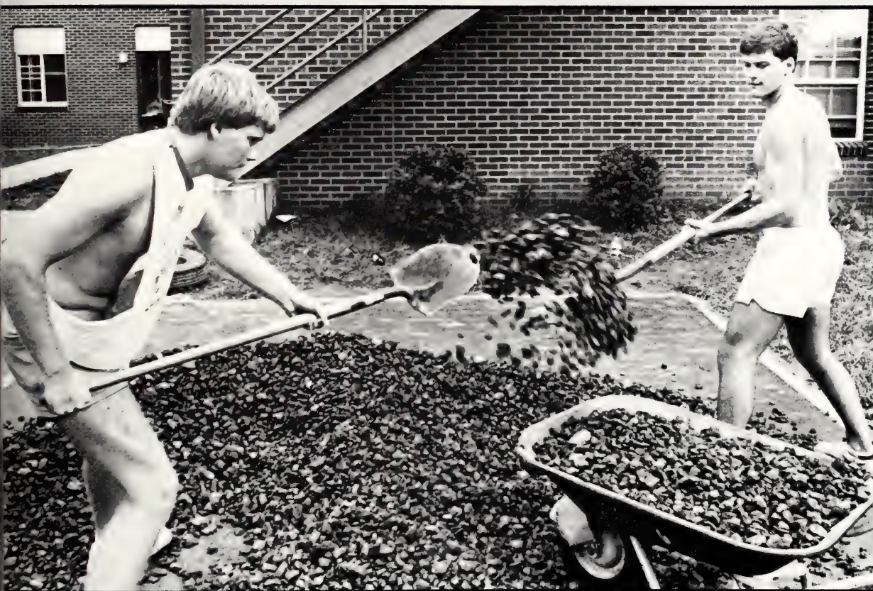
Jim Hill and Kevin Mott shovel building-rock while helping landscape the Sigma Chi house. (Photo by Jim Dietz)
