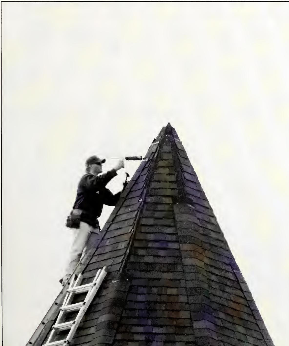
A construction worker puts finishing touches on a roof peak located on top of Fairchild Hall Dec. 3. (Photo by Ivan Kozar)
