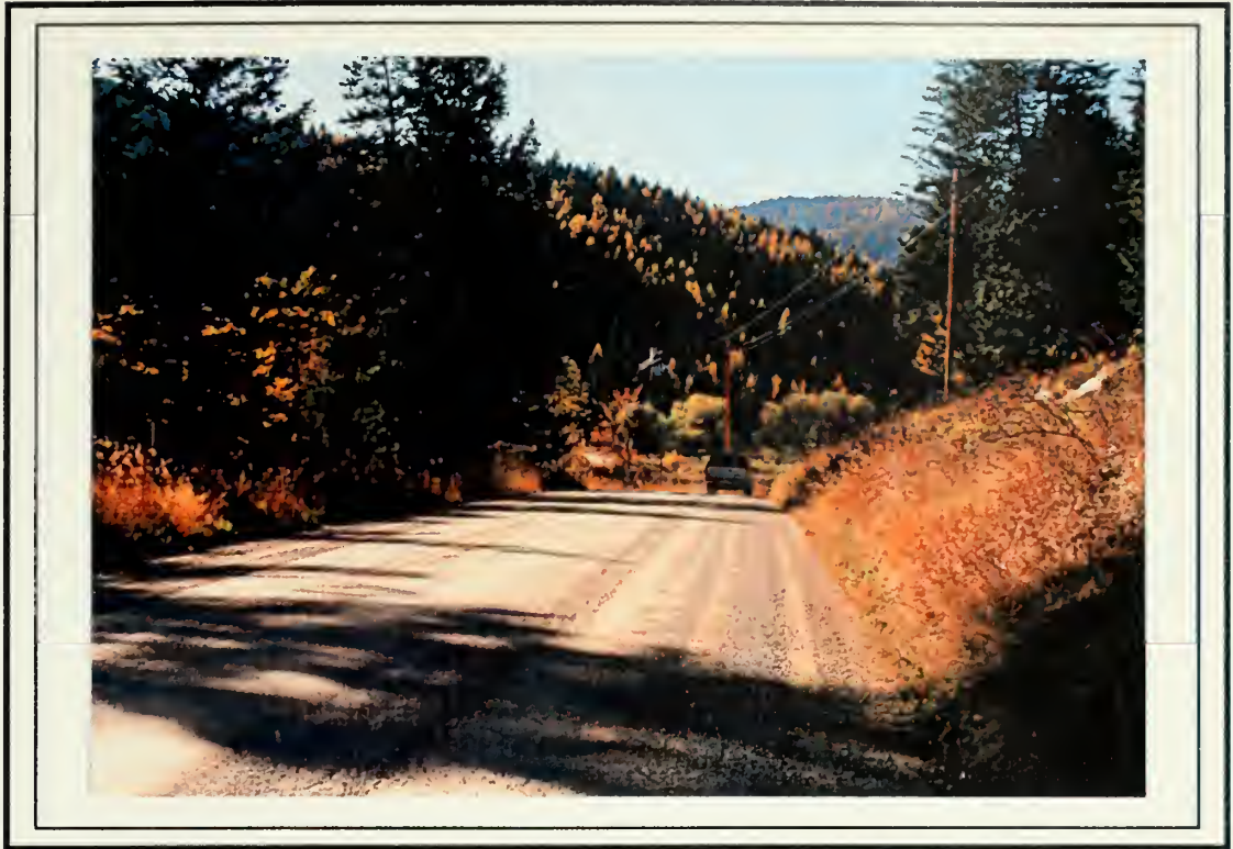
Mid Foys Canyon Road looking southeast
