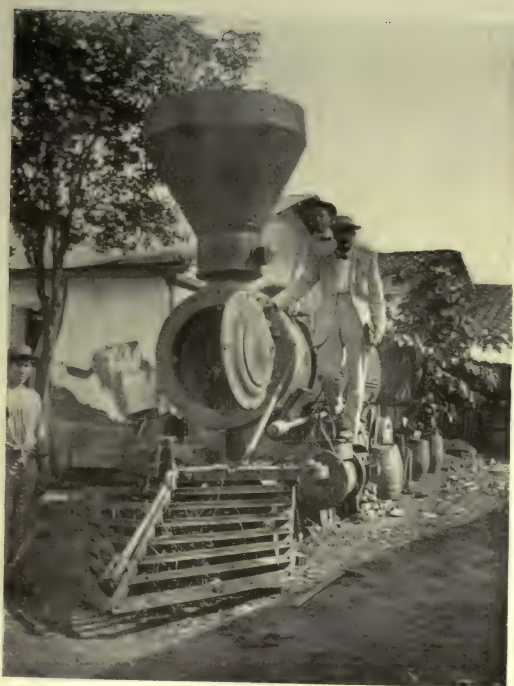
THE ENGINE "COLONEL CHURCH" ABANDONED BY RAILWAY ENGINEERS IN 1880
