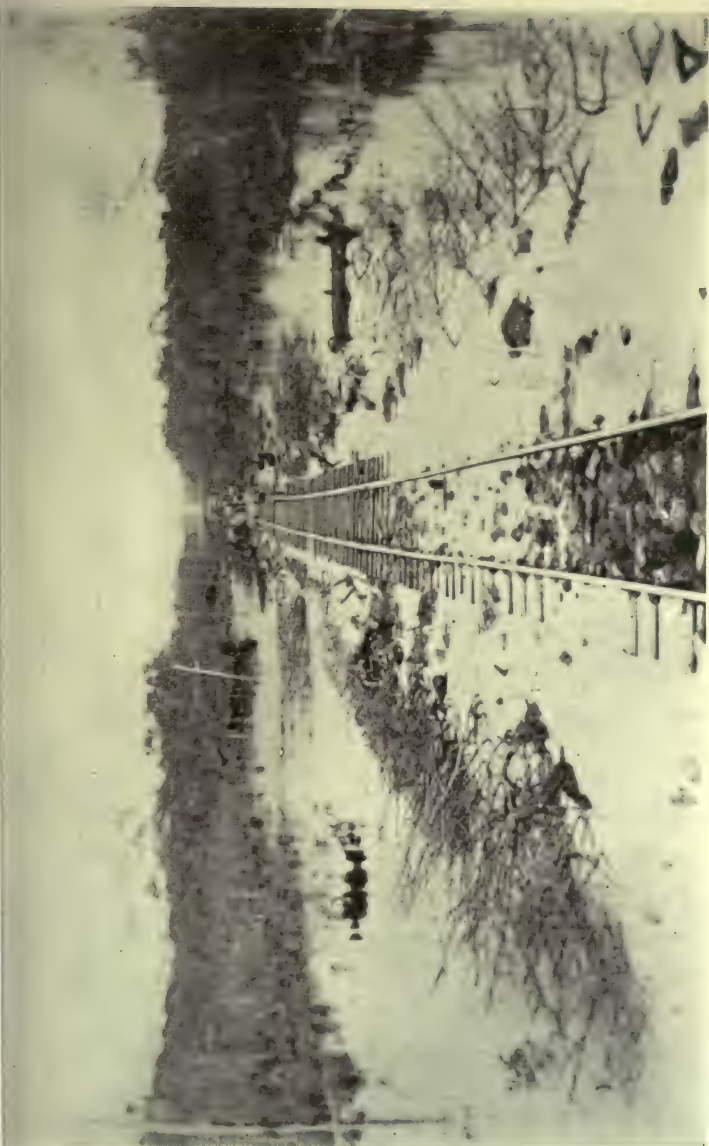
DIFFICULTIES OF RAILWAY CONSTRUCTION—RUNNING THE METALS THROUGH SWAMP ON CUT BRUSH FILLED UP WITH EARTH
